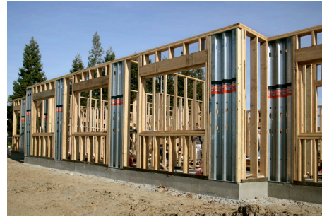
Example of a timber frame construction with Steel Strong-Wall™
