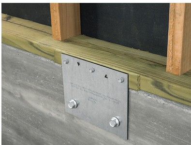
Reinforcement of the connection with the foundation
