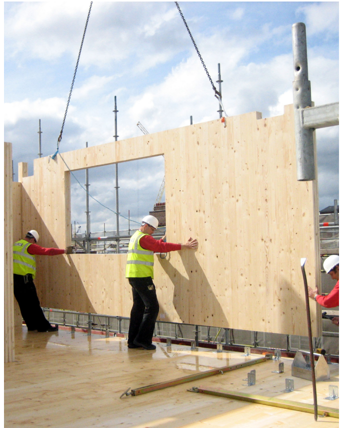
Stadthaus, Murray Grove. Image provided by KLH UK.
